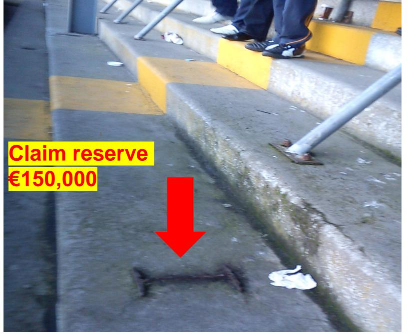
Could have been avoided if barrier footprint was fully removed when replaced
